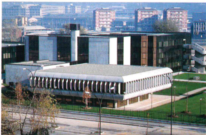
The complex of buildings forming the new « Lingotto » civic centre in Turin: modern architecture serving the collectivity and comprising social, medical and cultural functions.
